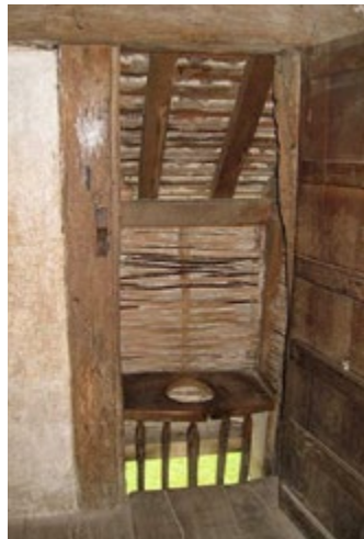
A 16th century garderobe, overhanging an outside wall. Wealden House, Sussex.
