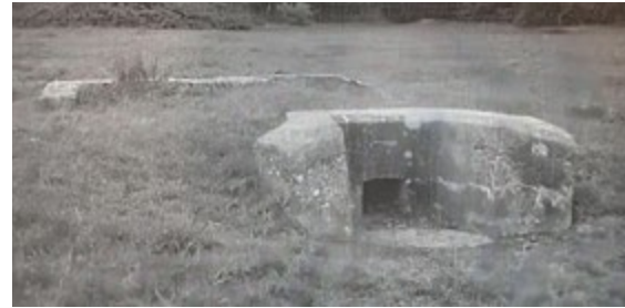
Disused water control on a former water meadow; a bridge for hay wagons.
